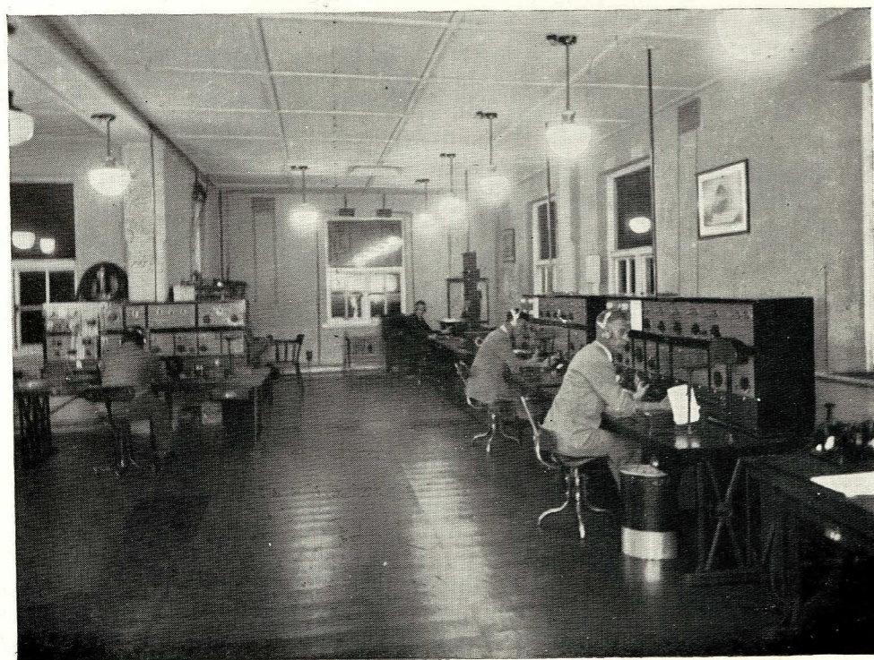
Further evidence of the complex organisation needed to deal with the radio traffic of the "QUEEN MARY" is afforded by these interior views at the Post Office shore stations at Portishead and Burnham. The upper view shows part of the equipment at Portishead. In the other picture operators are seen handling ships' radio messages at Burnham.
