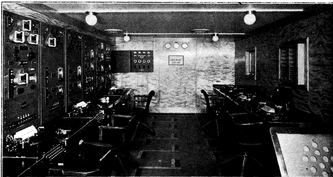
Occupying the centre of the receiving room are the operators desks and each has two receivers covering the full band of wavelengths in use.
